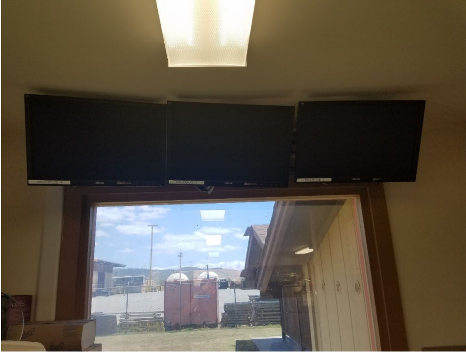
Photo 34: Existing security surveillance camera flat screen monitors to remain.
