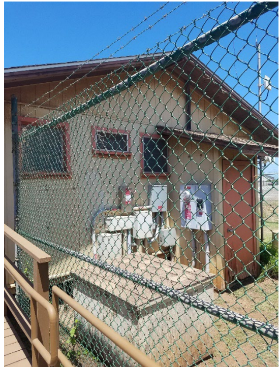
Photo 40: Existing water heater closet.
