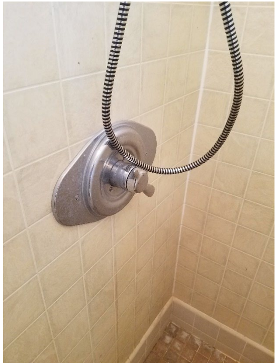
Photo 48: Existing shower mixing valve.
