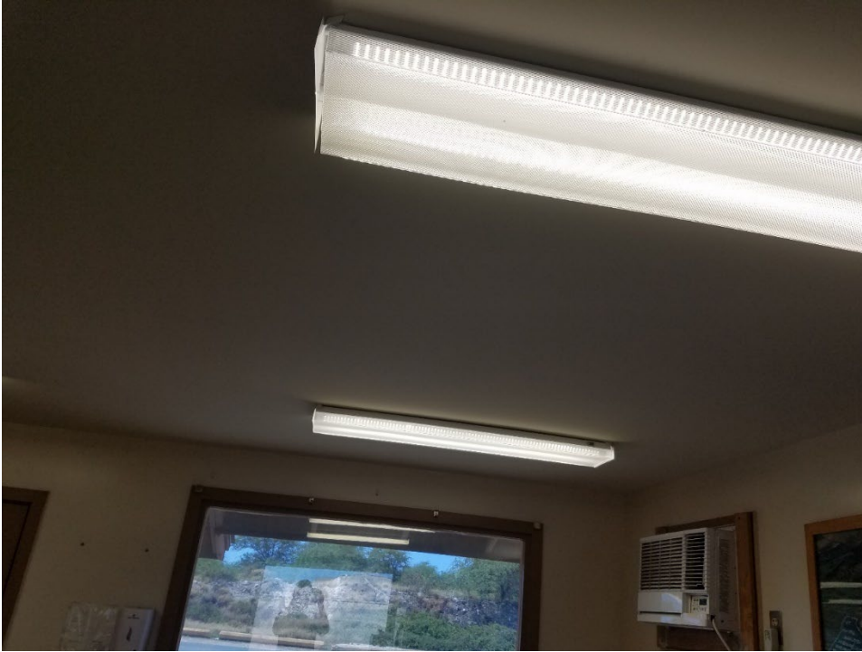
Photo 14: Office ceiling facing entry.
