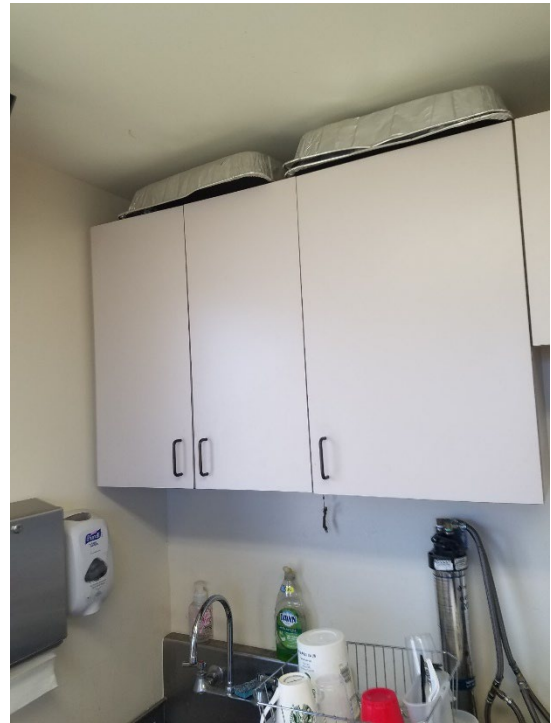
Photo 36: Existing wall mounted upper cabinets.
