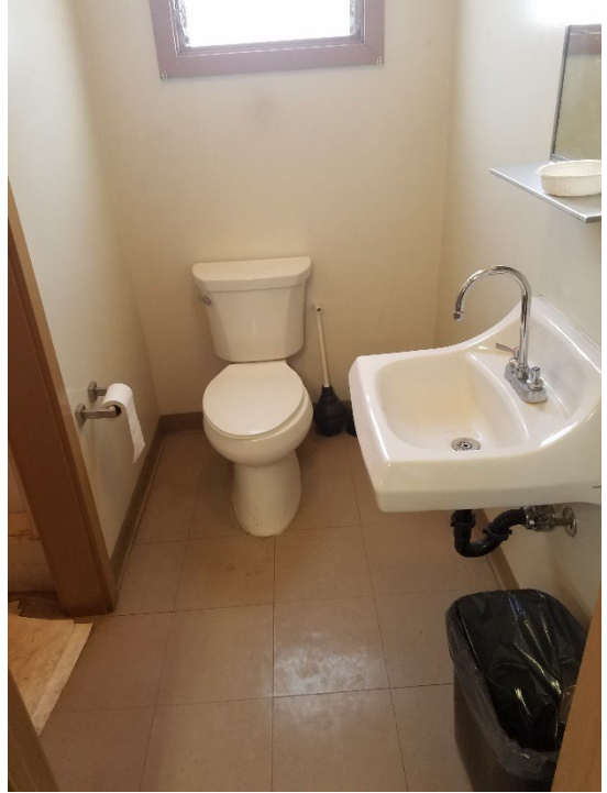
Photo 42: Existing water closet.
