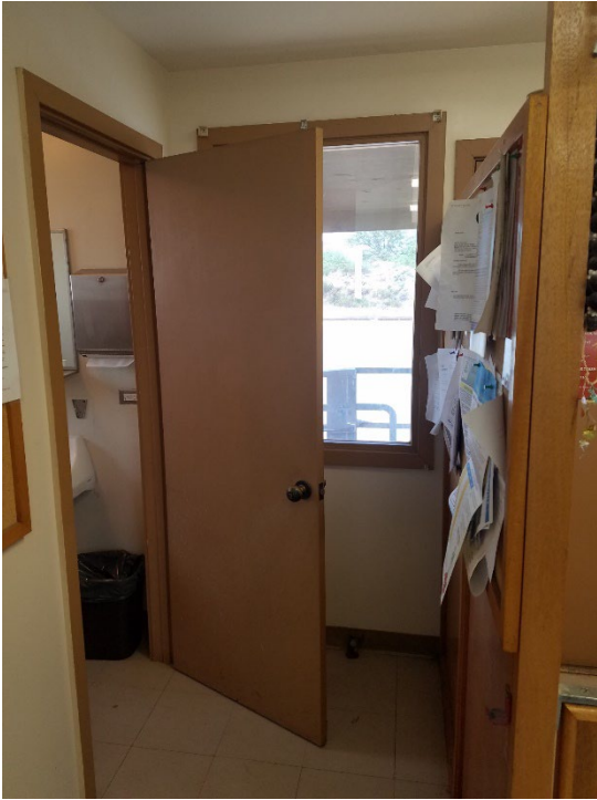
Photo 1: Entry to existing restroom.
