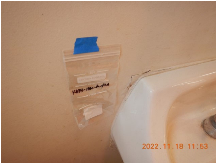
Photo 27 - KBPH-M-03A (Close-up) [BB\DSCN0020.JPG]
