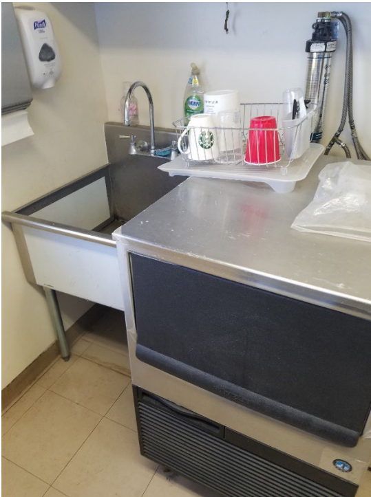
Photo 35: Existing scullery sink and ice maker.
