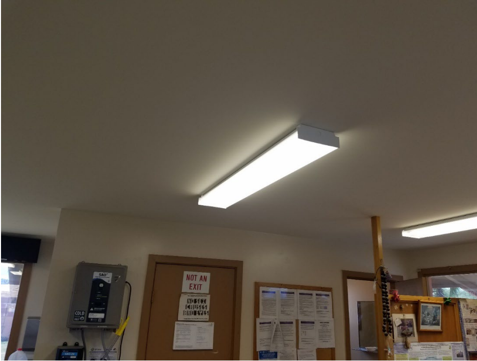
Photo 12: Office ceiling facing janitor/electoral closet and restroom.
