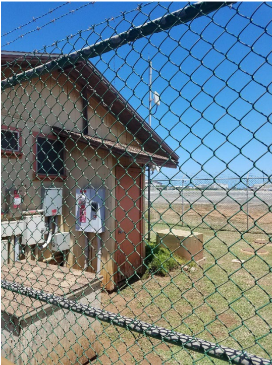
Photo 39: Existing water heater closet.
