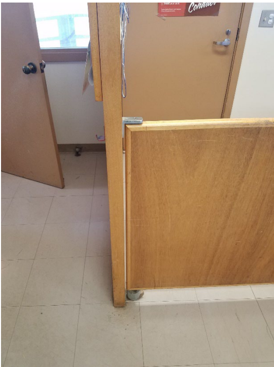
Photo 7: Gate - office side.
