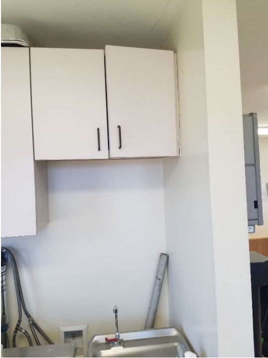
Photo 37: Existing wall mounted upper cabinets.
