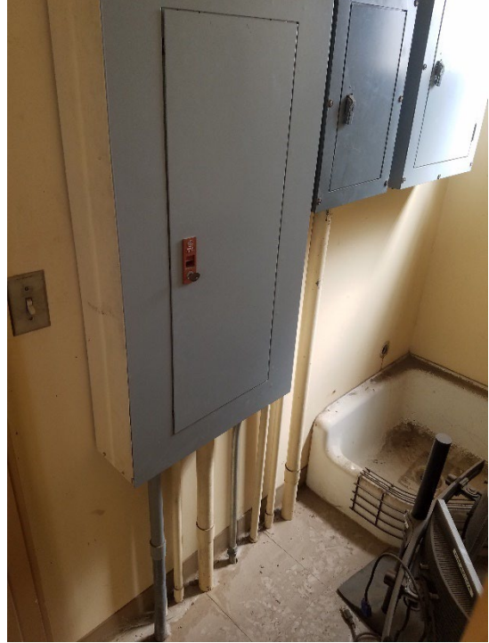
Photo 45: Existing janitor/electrical closet.
