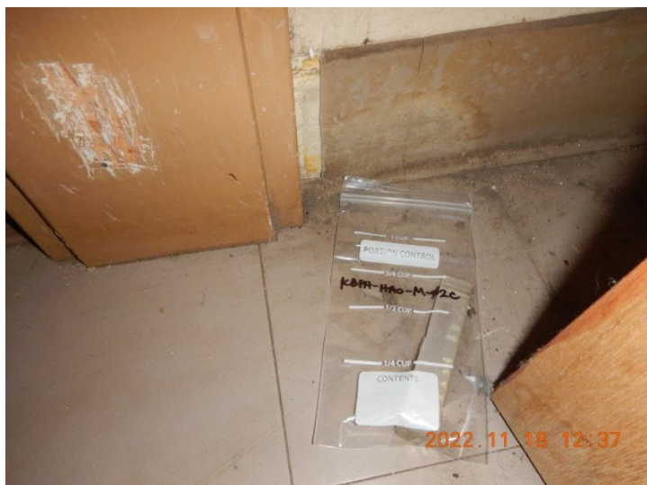
Photo 25 - KBPH-M-02C (Close-up) [AL\DSCN8395.JPG]
