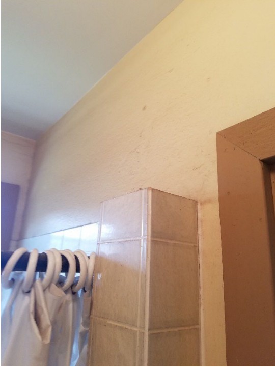
Photo 40: Existing shower at wall.
