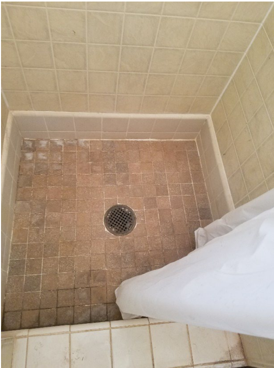
Photo 47: Existing shower drain.
