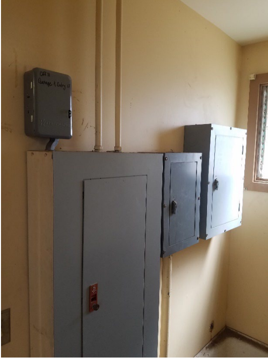
Photo 44: Existing janitor/electrical closet.
