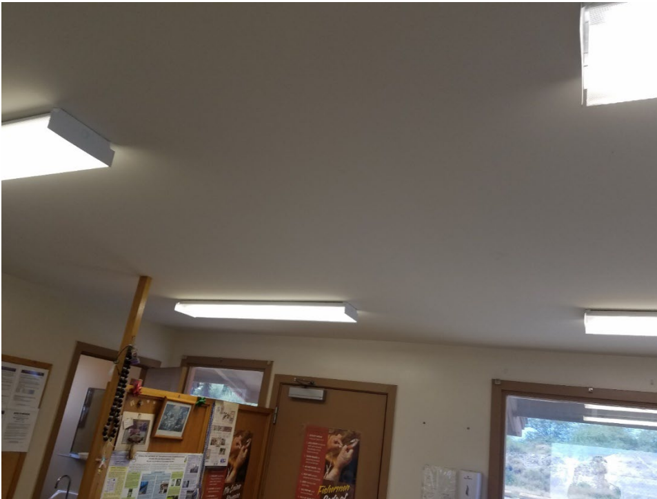
Photo 13: Office ceiling facing entry.
