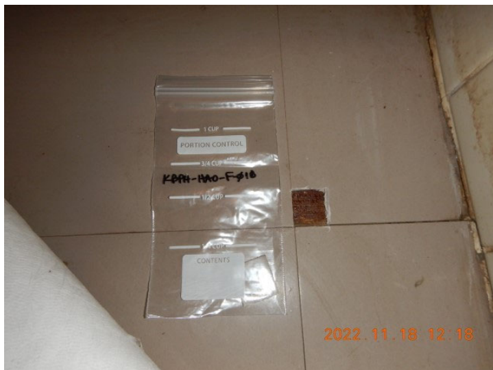
Photo 3 - KBPH-F-01B (Close-up) [AL\DSCN8387.JPG]
