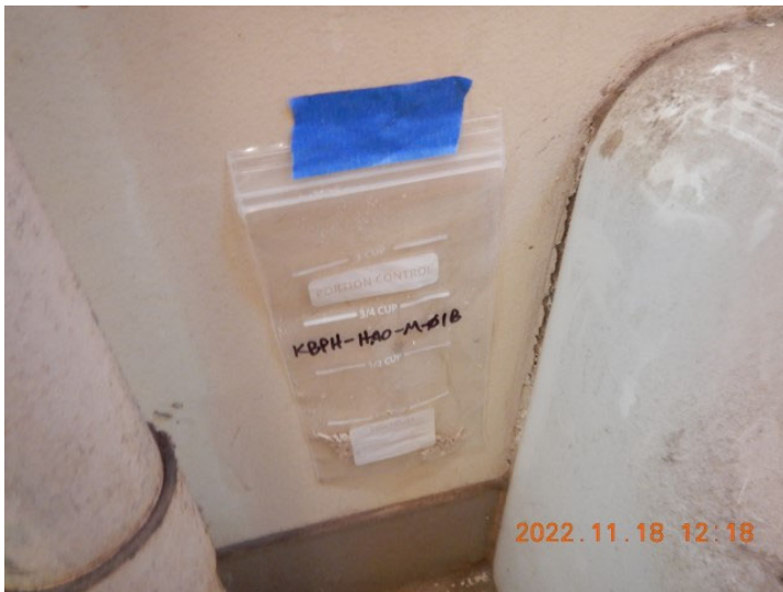
Photo 20 - KBPH-M-01B (Close-up) [BB\DSCN0027.JPG]
