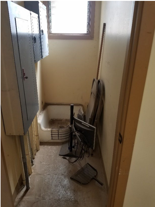
Photo 42: Existing janitor/electrical closet.
