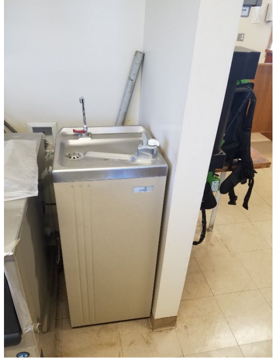
Photo 38: Existing drinking fountain.
