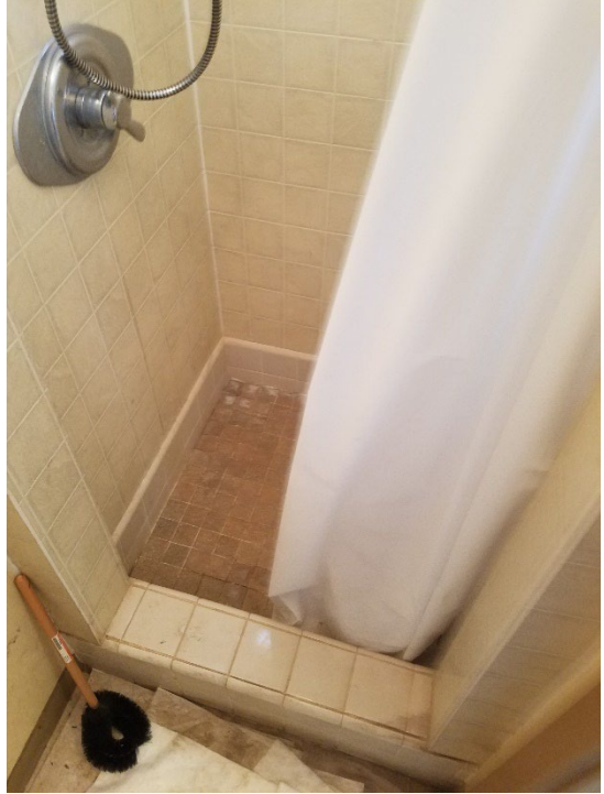
Photo 46: Existing shower curb.
