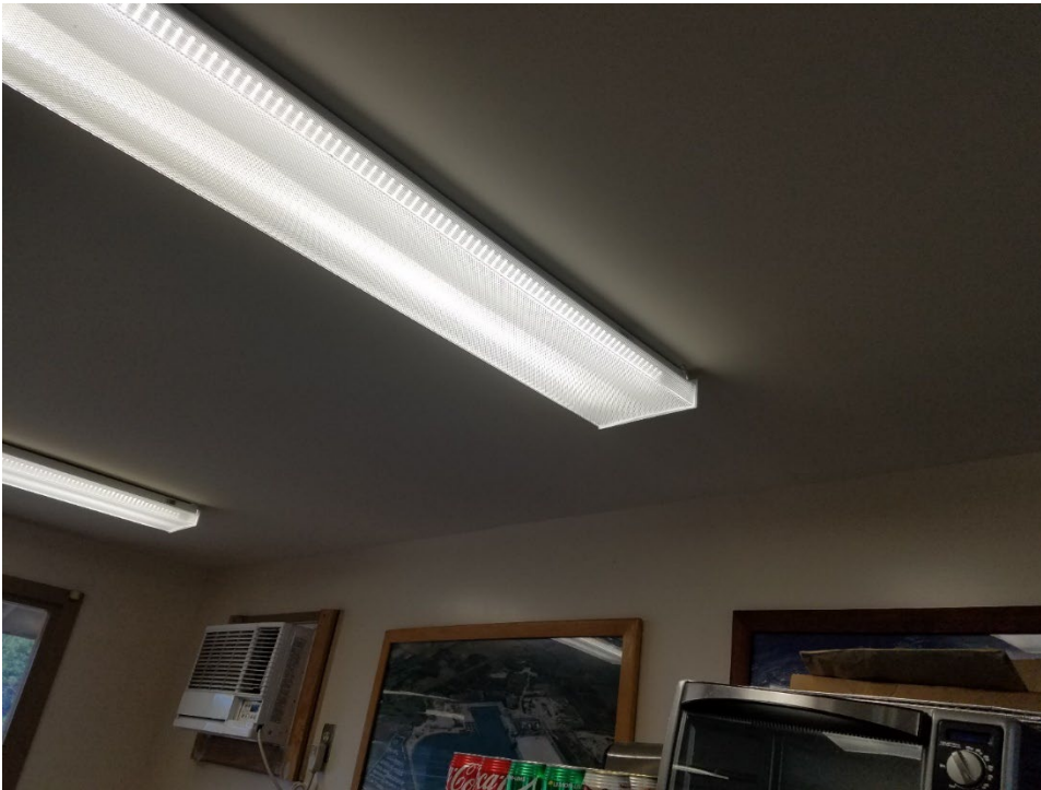
Photo 15: Office ceiling facing entry.
